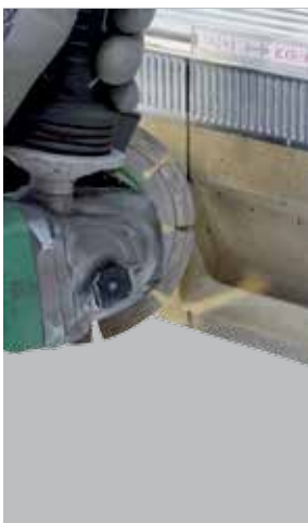
cutting the channel body to size
